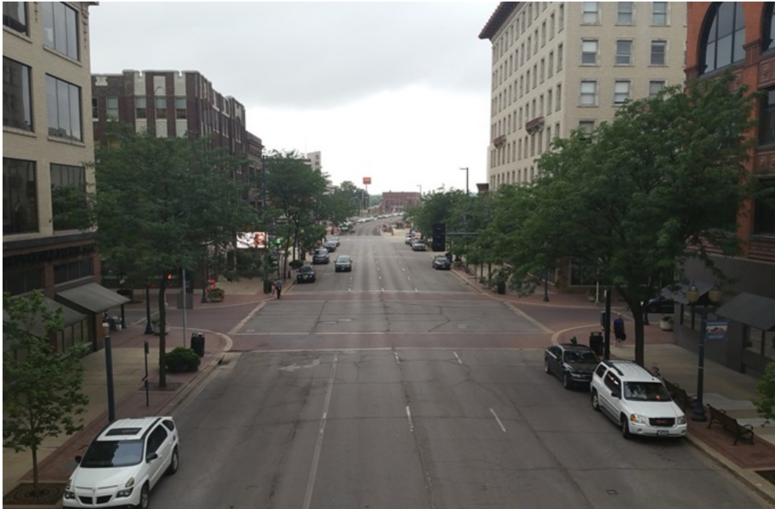
A typical street in downtown Cedar Rapids before and after conversion from four-lane one-way to two-lane two-way with buffered cycletrack.
