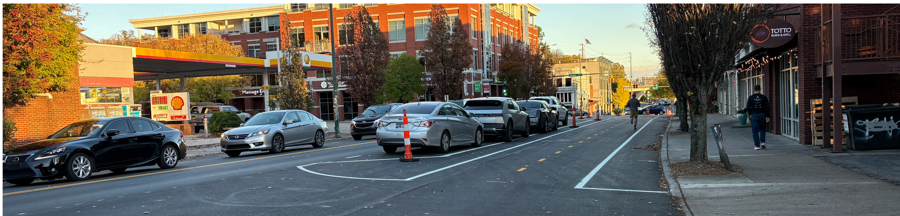
Before and Interim: awaiting final paint and planters, the street reconfiguration replaces two excess driving lanes with parallel parking, a cycle track, and an expanded walking zone.
